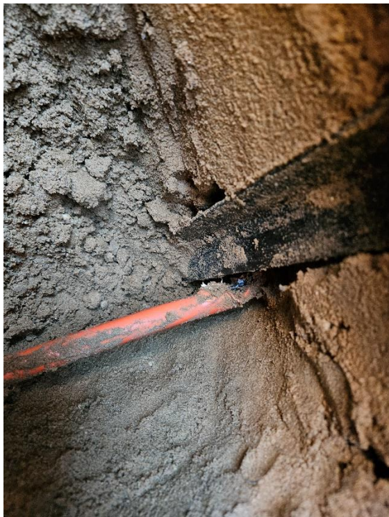
Cable slab removed showing star picket impact with streetlight cable.
