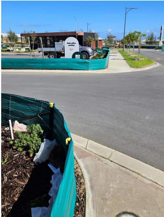
Star pickets installed along footpath within EVE power cable alignment.
