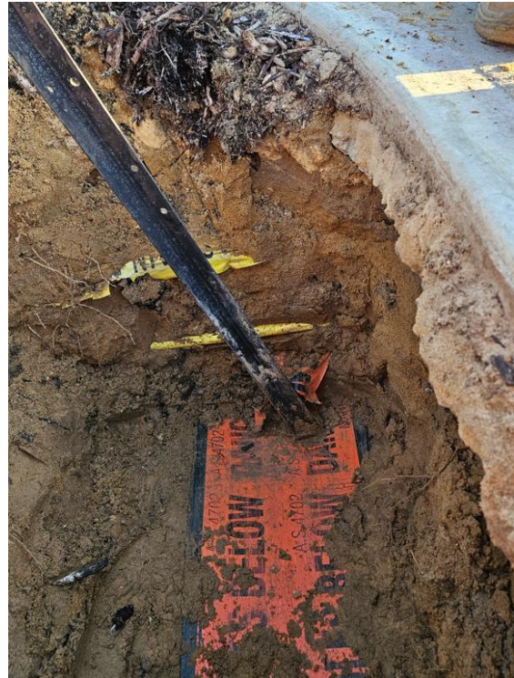
1800mm star picket driven through cable slab. Star picket also narrowly missed the gas service.
